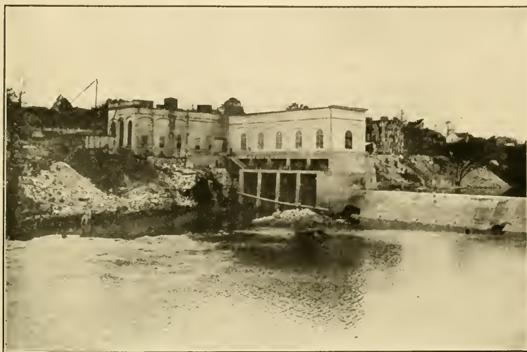
Fig. 394.—Hydroelectric power plant at Williams.
